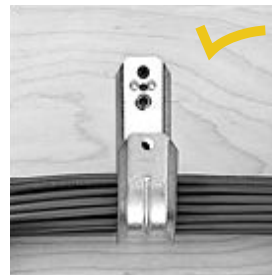
Use j-hooks or similar devices designed to support cables.
