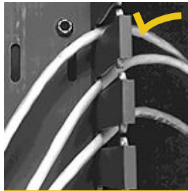
Use sweeping bends, no tighter than the curve of a Coke can.
