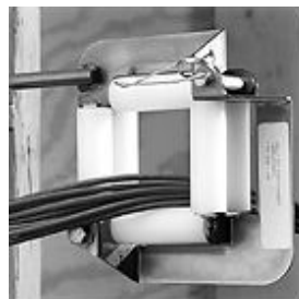
Use a cable pulling accessory.
