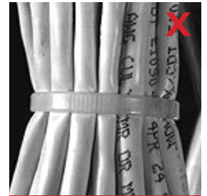
Do not overstress cables by over tightening cable ties, especially to the point where crush-stress is visible.
