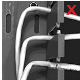
Bend ratio = 4x diameter. Don't allow the cable to form right angles or sharp bends.
